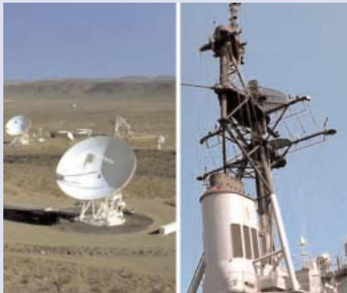
Left: Antennas at Goldstone Deep Space Communications Complex (part of NASA's Deep Space Network) help provide radio communications for NASA's interplanetary spacecraft. Right: Surface search radar and air search radar are mounted on the foremast of a guided missile destroyer. Photo courtesy NASA (left), Department of Defense (right)
