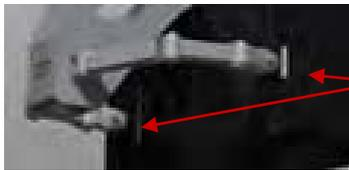
**Brackets can be fixed using nuts and bolts. This allows the screens to be replaced if needed.**
